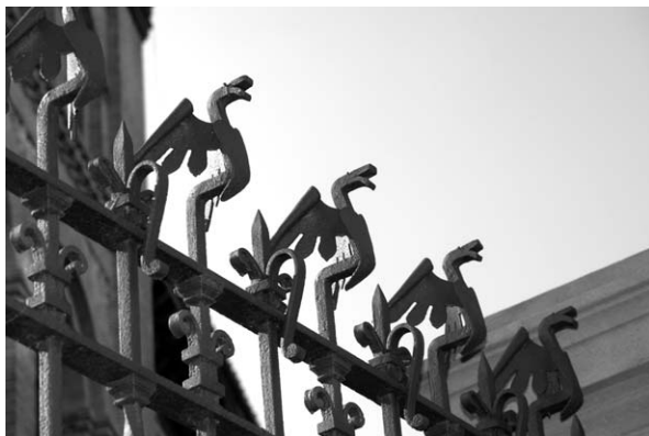
Fig. 9. Tops of the railings of the former building for the Faculties of Medicine and Sciences in Zaragoza (Calle del Doctor Cerrada).
