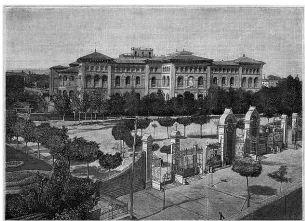
Fig. 3. Aspect of the former building for the Faculties of Medicine and Sciences in Zaragoza when inaugurated (wood engraving of T. Capuz made from a photograph in Anon (1893a), p. 1, and published in Reparaz (1893), p. 285).
