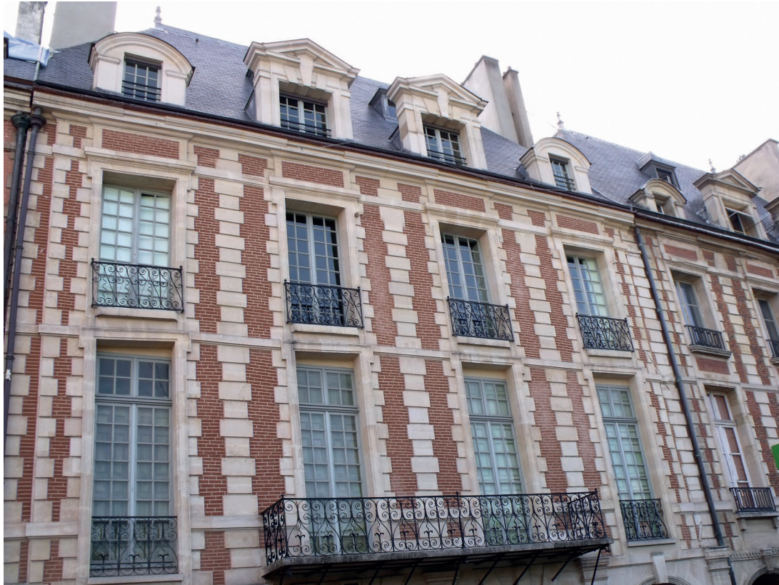
FIG. 16. — Residence of Deshayes at 20 place des Vosges, Paris 4 ème arrondissement.
